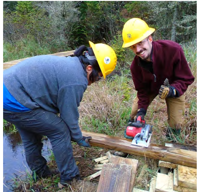
Student Conservation Association staff replacing a boardwalk in the Adirondacks
