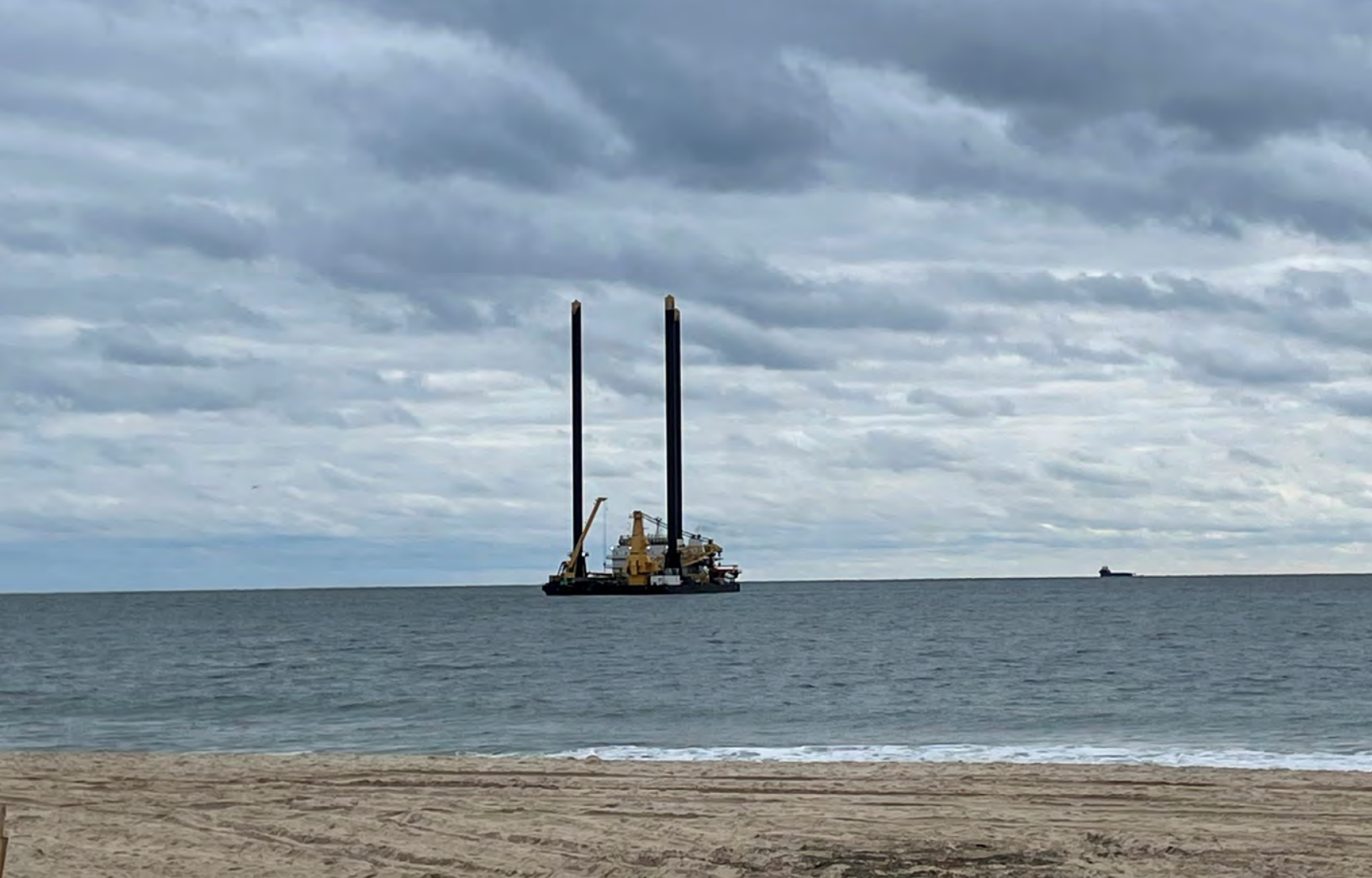
Long Island South Shore wind construction
