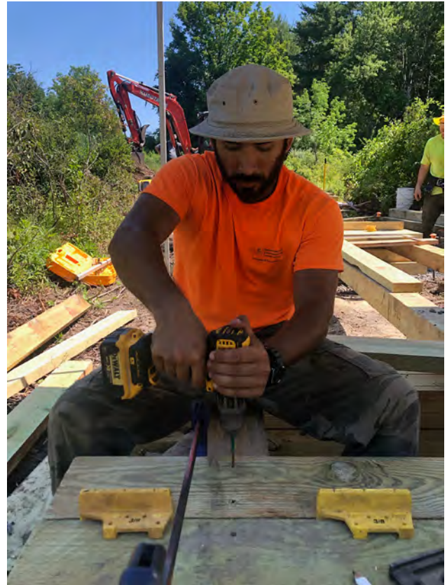
Construction of the new Fisher Trail at Five Rivers
