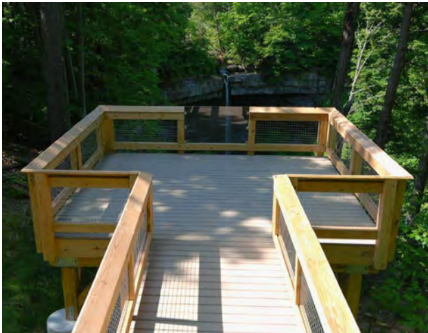
New viewing platform at Carpenter Falls Unique Area
